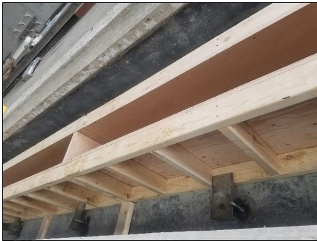
Fig 6.1. Side panels of formwork
