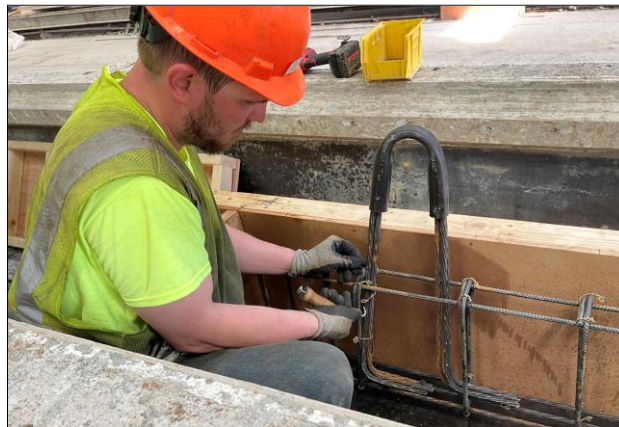
Fig 6.7. Transport hook
