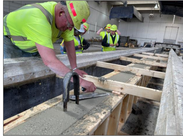
Fig 6.9. Finishing the concrete beam surface
