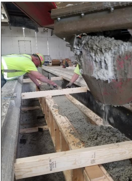
Fig 16.4. Concrete pouring and finishing operation
