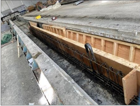
Fig 6.5. Completed rebar cage
