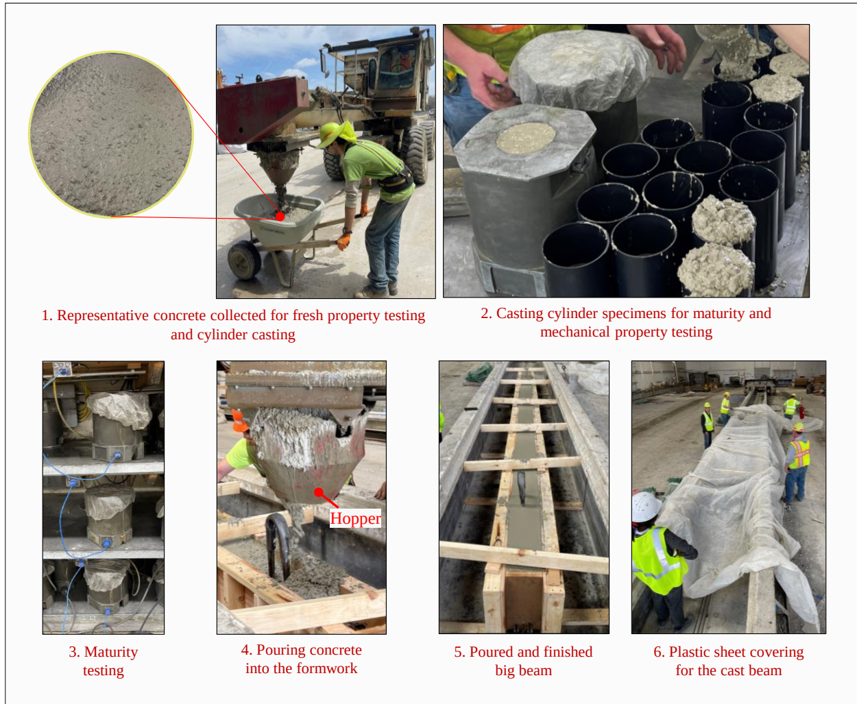
Fig 6.12. An overview of tasks performed at the concrete plant
