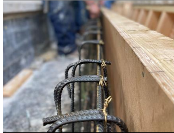
Fig 6.6. Stirrup tie down
