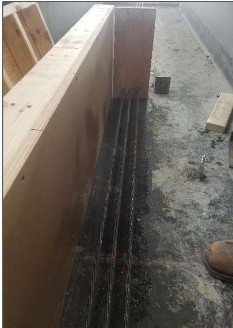
Fig 6.3. Prestressing strand through end panel
