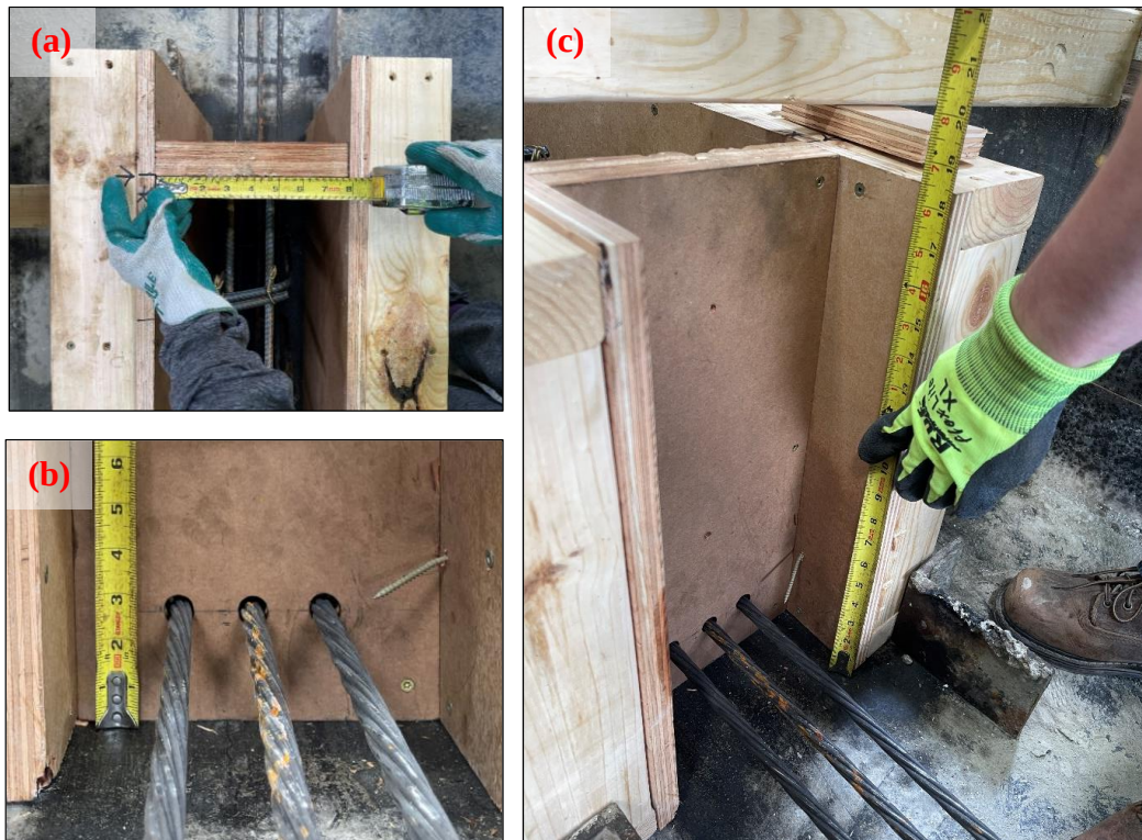
Fig 16.2. Measurement check for the formwork dimensions
