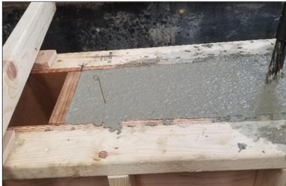
Fig 6.10. Identification tie placed at right end of the beam
