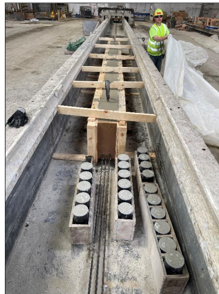
Fig 16.5. Casted beam and cylinders
